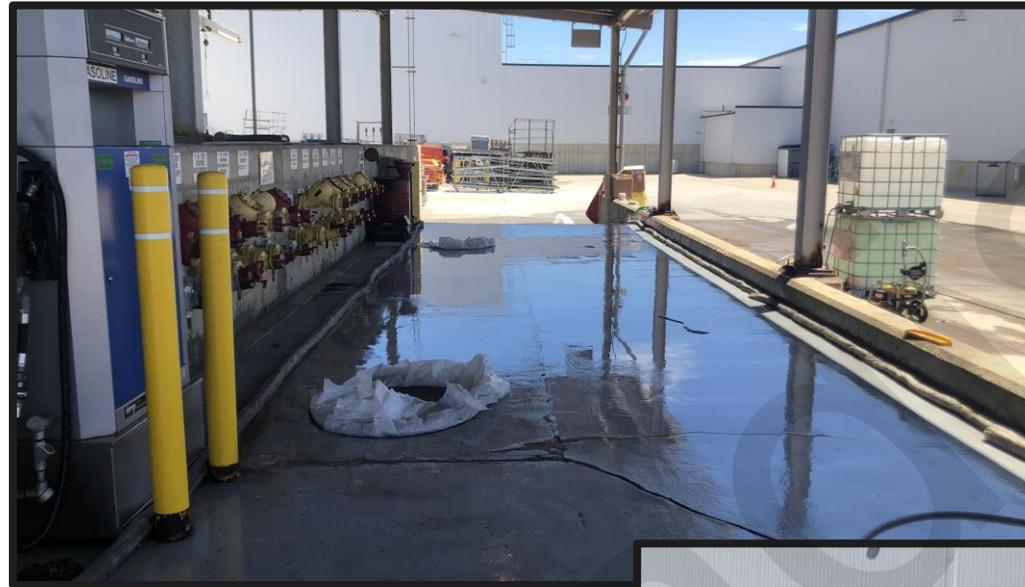
Arcadis cleaned subsurface vault with Fluoro Fighter™ - used 825 gallons of cleaning agent over two days
